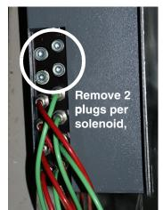
Fig. 10: Outlet Ports
