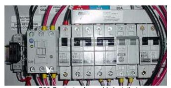
C30 Contactor Assembly Installed
